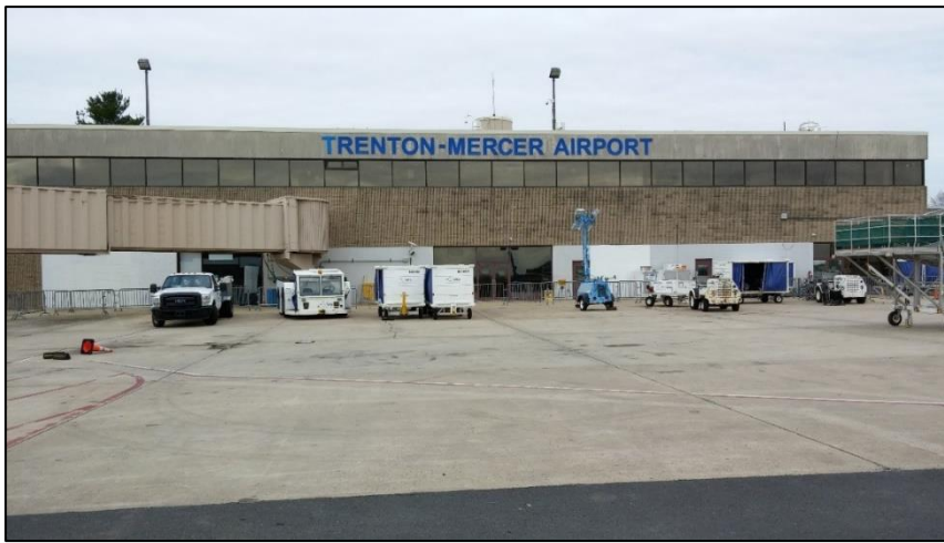
Photo 5: View of terminal building from apron (Date: April 2015)
